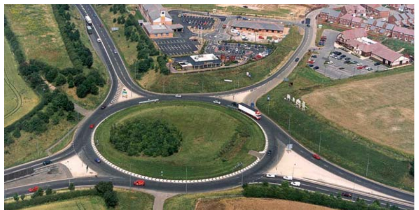
A45 Roundabout, Wilby and Associated 100 acre Development
