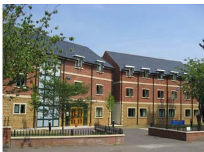
Student Accommodation, Uppingham School
