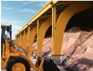
A14 Maintenance Depot
