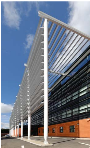
Stevenage Police Station
