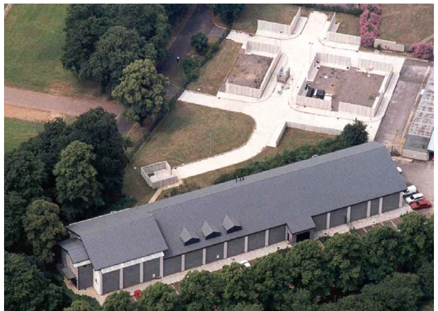
Police Firearms and Public Order Training Centre, Northampton
