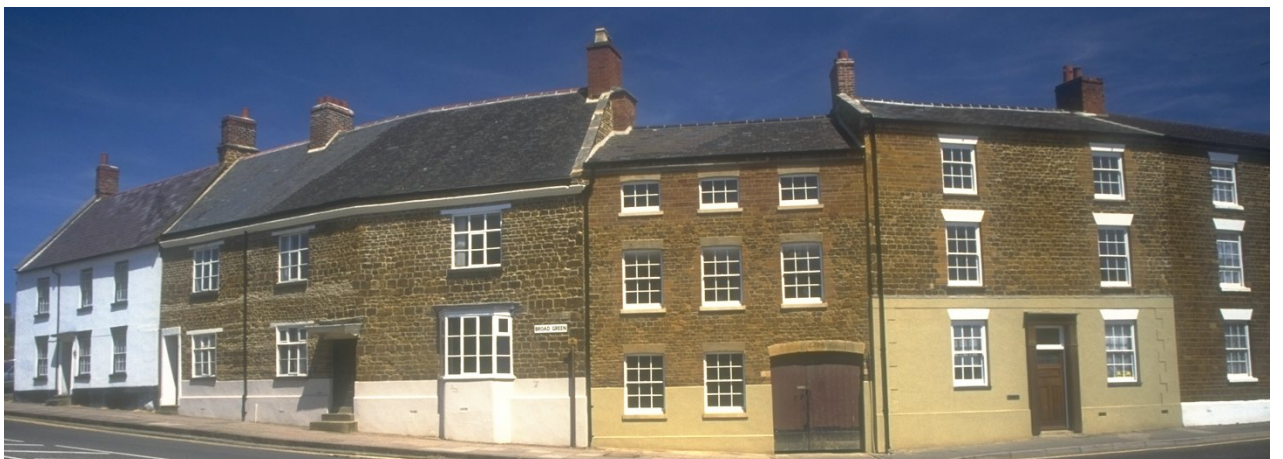
Office Restoration - Wellingborough
